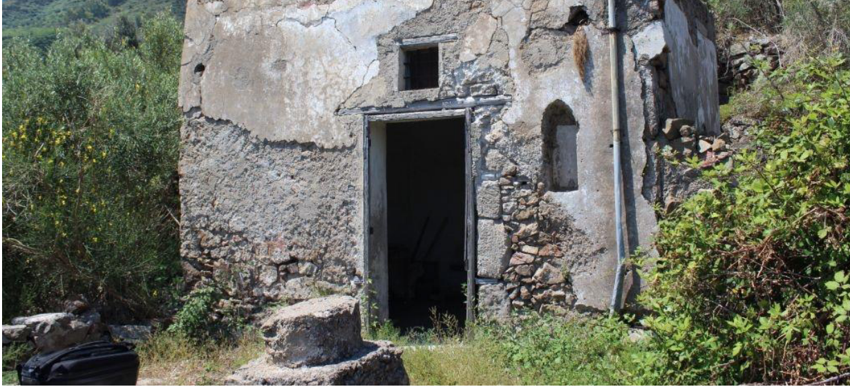
Figure 14. The traditional plaster: lime mortar and fine lapilli
