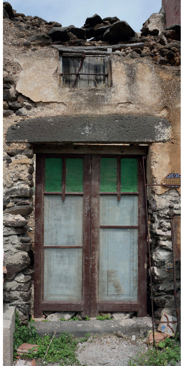
Figure 6. Main entrance of the case study building
