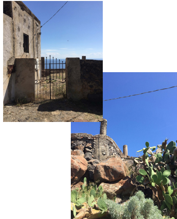
Figure 5. Terrace and current condition
