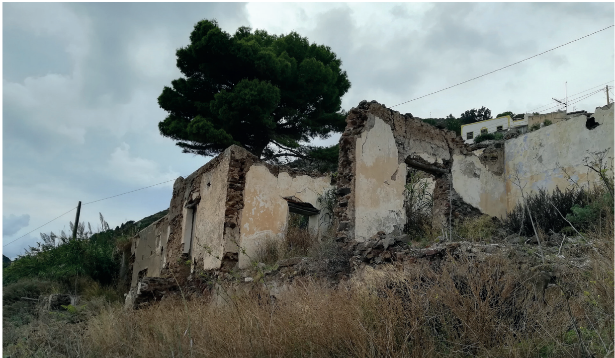
Figure 10. Existing conditions of the case study building
