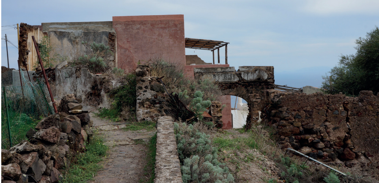
Figure 7. Picture of the case study building (west view)
