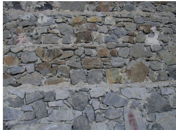
Figure 11. Rough-hewn stones and horizontal “courses” of lime mortar
