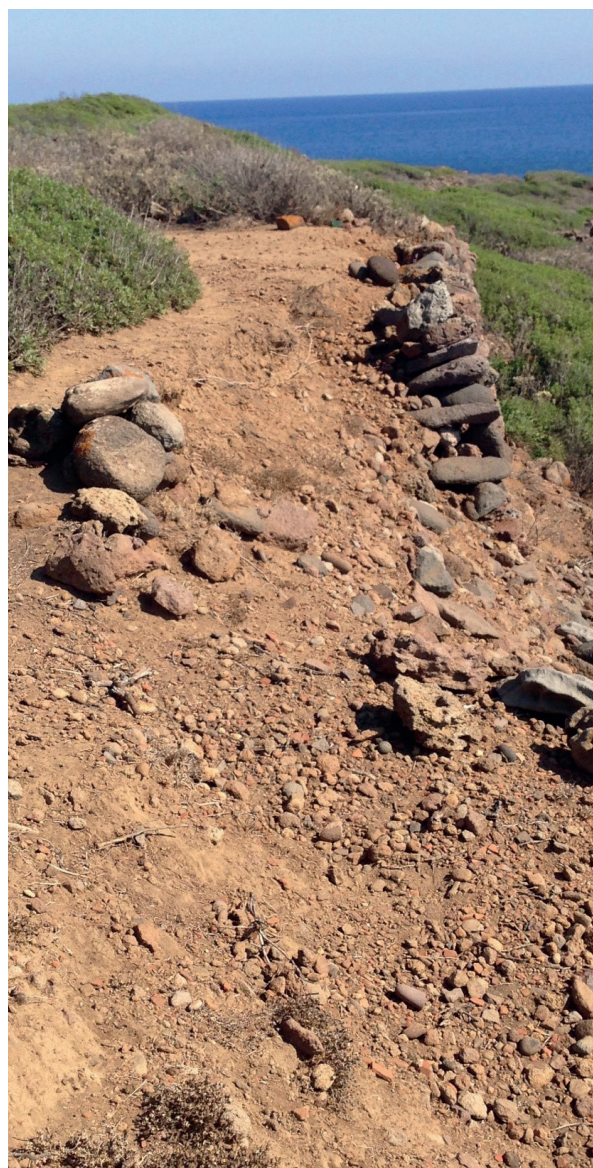
Figure 2. An example of collapsed dry-stone wall in the Island of Filicudi. (Photo by A. Sardella)
