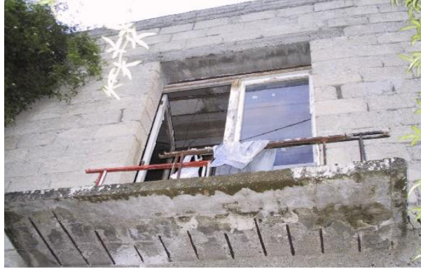
Prefabricated joists and hollow clay blocks floor
