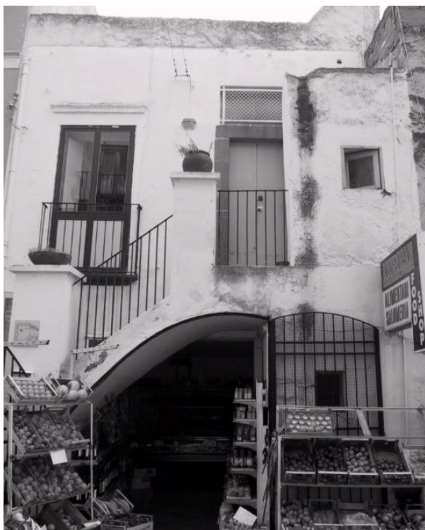
Figure 13. Typical staircase (exterior and internal)
