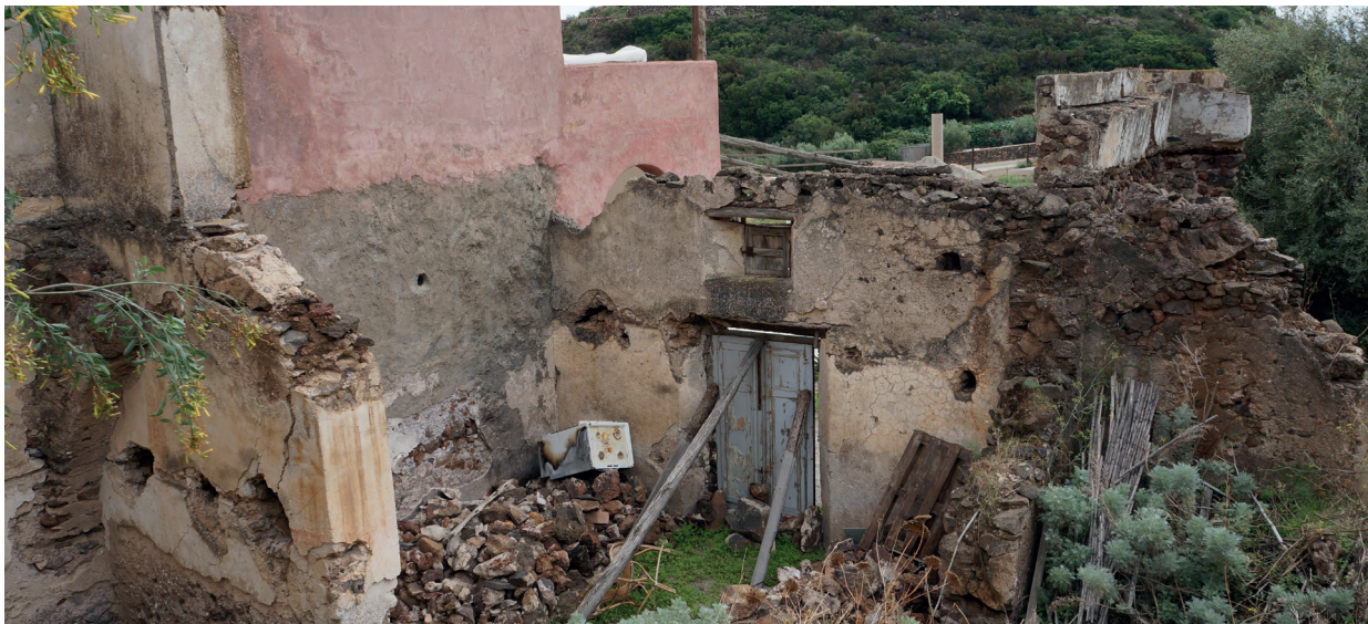
Figure 8. Existing conditions of the case study building
