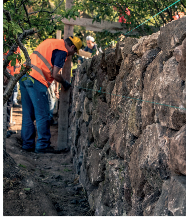
Figure 5. Final phase: layering and levelling phases. (Photo by G. Taranto)
