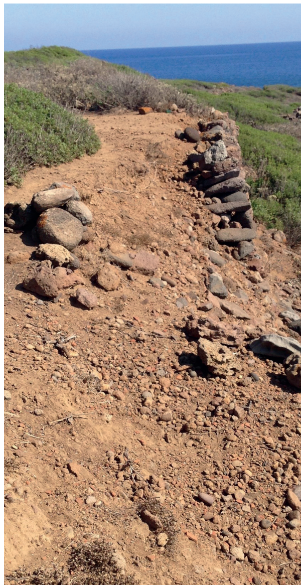
Figure 2. An example of collapsed dry-stone wall in the Island of Filicudi. (Photo by A. Sardella)
