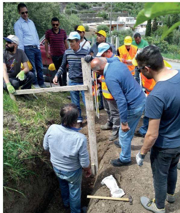
Figure 3. Master builders showing how to prepare guides for regulating the slope of the wall before its construction (Photo by A. Sardella)
