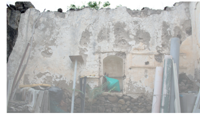
PLACEMENT OF THE LAST PLASTER LAYER
