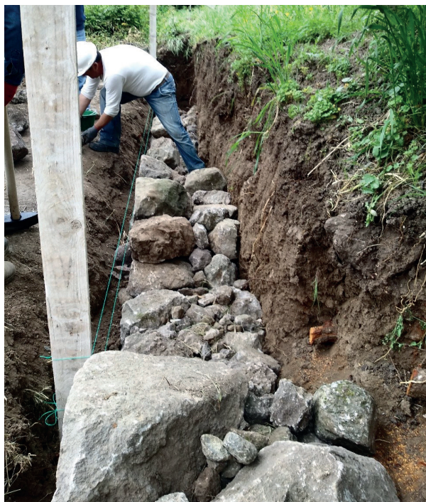
Figure 4. Practitioners positioning the drainage internal filling of the wall with smaller stones. (Photo by A. Sardella)
