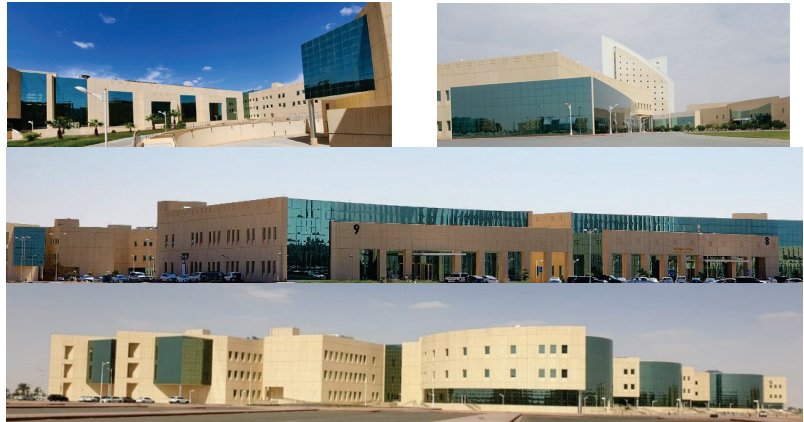
Figure 1. Exterior views of certain Najran University buildings highlighting glazed facades.
