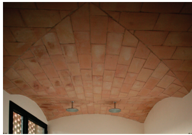
Figure 1. Traditional tile vault.
