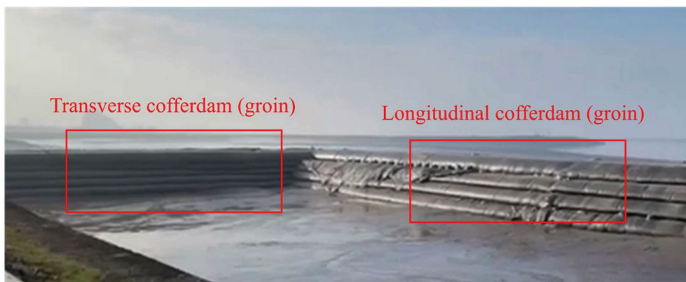
Figure 1. Transverse cofferdam and longitudinal cofferdam.
