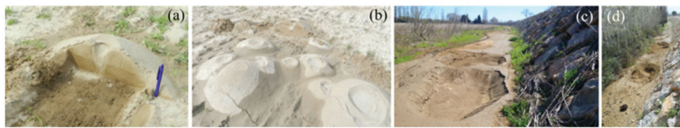
Figure 1. (a,b) Sand boils in the protected area, (c,d) Sinkholes observed around the levee toe.
