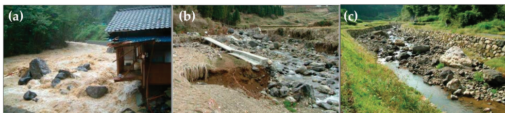
Figure 2. The river under study: (a) the river during the flood of 2005; (b) the river after the flood of 2005; (c) the river after restoration in 2009.
