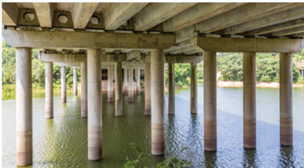
Figure 1. A group of bridge piers.
