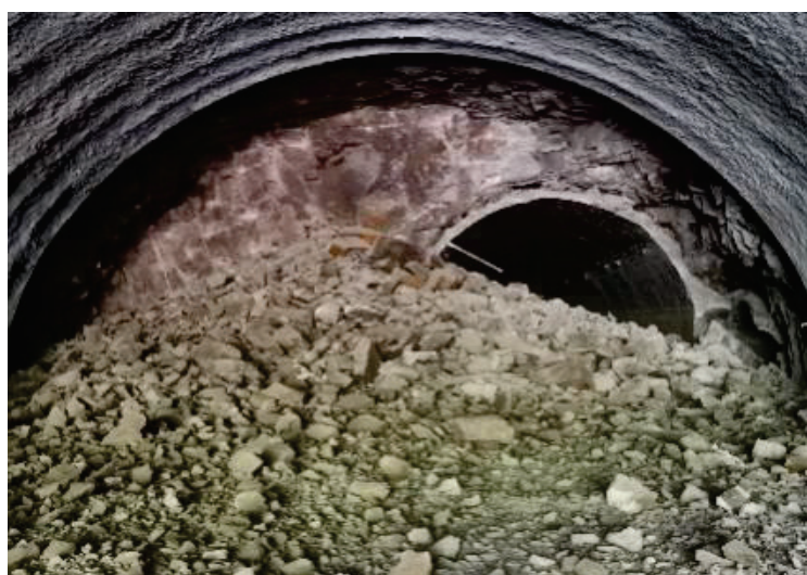
Figure 19. The upper part of NK18+110 section before and after expansion.
