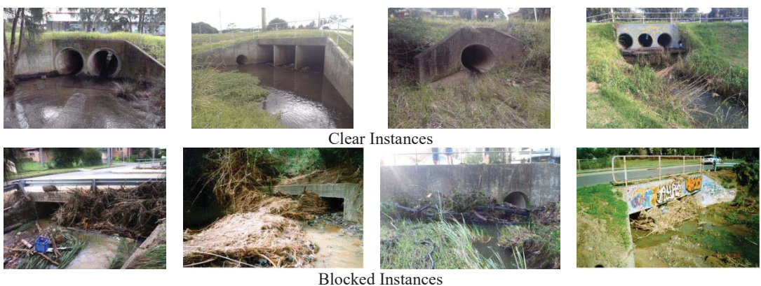
Figure 1. Sample instances of clear (First row) and blocked (Second row) culverts from ICOB.
