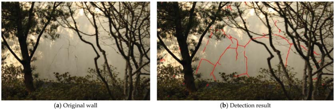
Figure 14. Detection of cracks on wall with interference factors.
