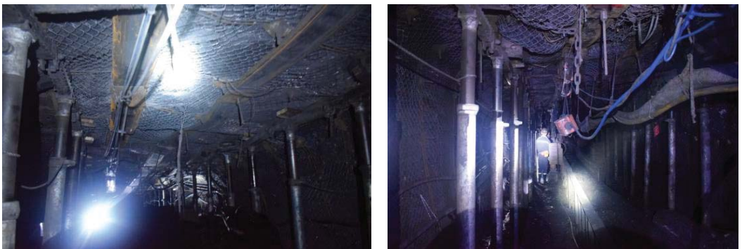
Figure 16. Effect of on-site advanced temporary support.
