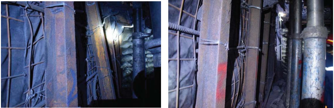
Figure 14. On-site retaining support effect.
