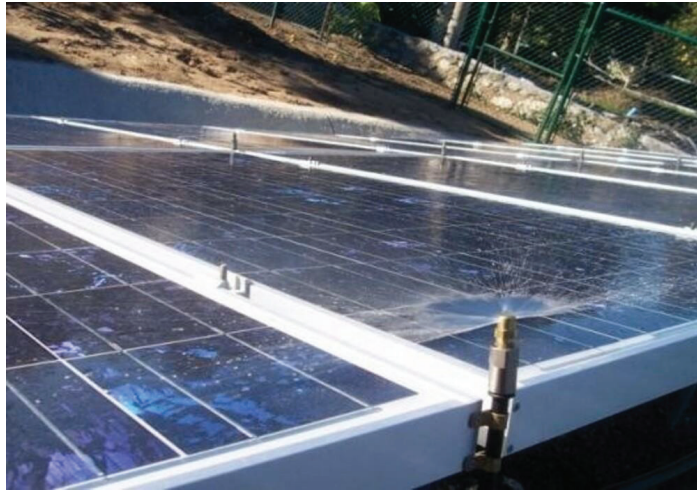
Figure 3. Demonstration of the heliotex method of cleaning solar panels [45].
