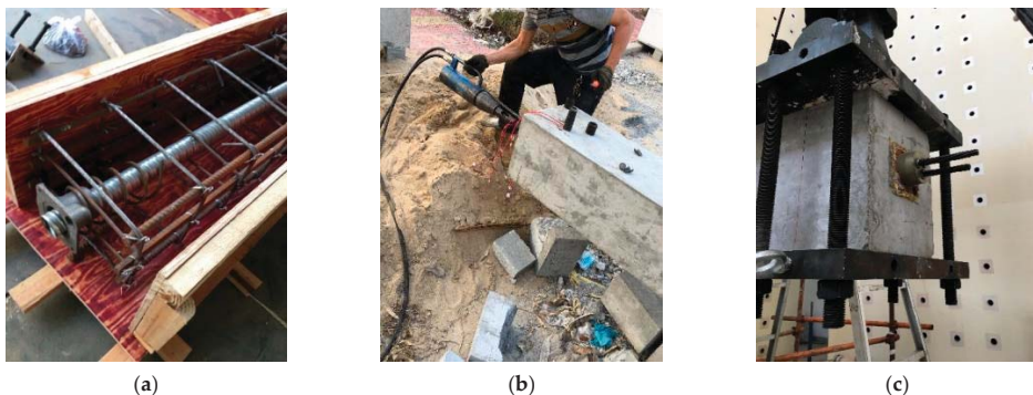
Figure 3. Post-tensioning tendon construction: (a) embedding corrugated duct; (b) prestress wire tensioning; (c) prestress wire anchorage.
