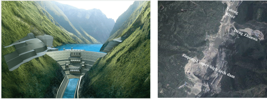
Figure 5. The simulation of the scenario and the of Jinping-I super-high arch dam.
