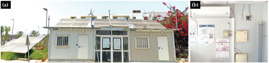
Figure 1. (a) Energy Efficient Building Lab (EEBLab) test site; (b) Interior side wall of EEBLab with ventilation fan and a set of sensors and other equipment.
