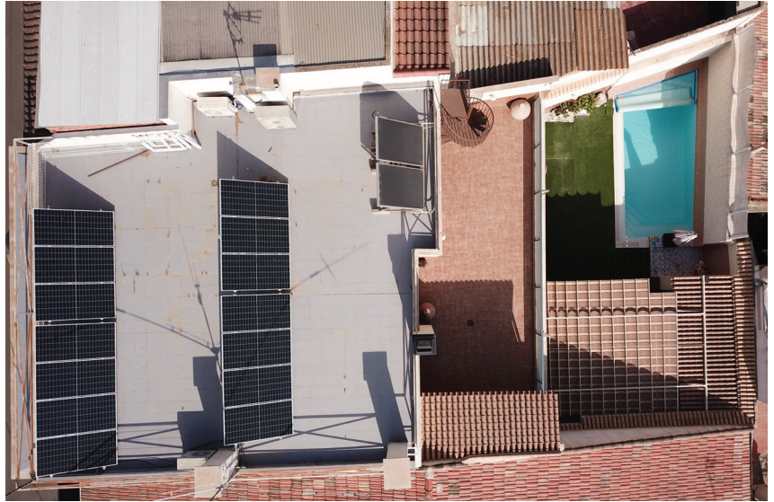
Figure 13. Aerial view of the test-bed location. Pool, PV panels, HVAC and heating units visible.
