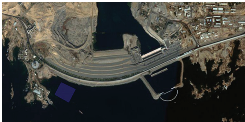
Figure 5. Location FPV system on Aswan High Dam covering 50,000 m 2 .
