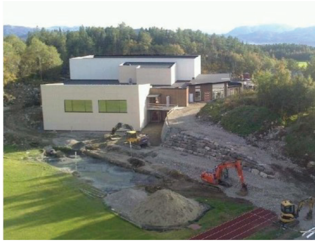
Figure 3. The northern façade of the building.
