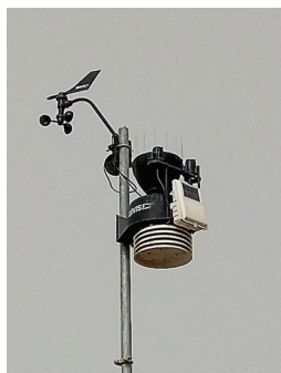
Figure 4. Rooftop Weather Station.
