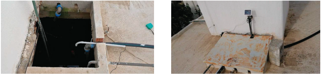
Figure 12. Measurement of the water level in a roof tank.
