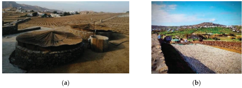
Figure 9. (a) Open top water tanks; (b) Sub-surface rainwater collection system.
