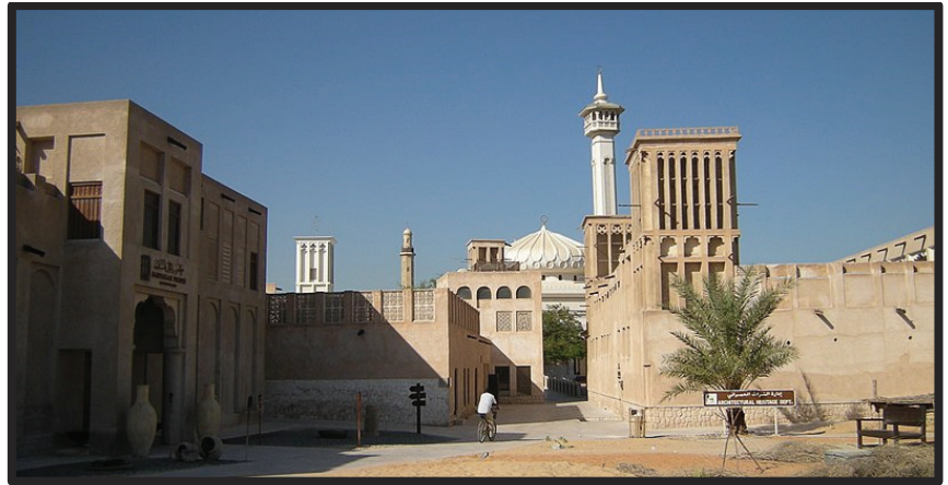
Figure 34. Four-Sided windcatchers in Bastakiya, Dubai, UAE. modified by authors, original photograph by Russavia under Creative Commons Attribution 2.0 Generic.
