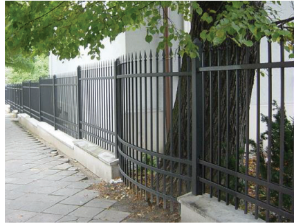
Figure 25. Planned lack of foundations to protect an ancient linden tree (photo M. Dudkiewicz, 2018).
