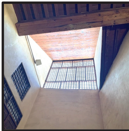
Figure 15. An interior view of the windcatcher of Bayt al-Suhaymi.
