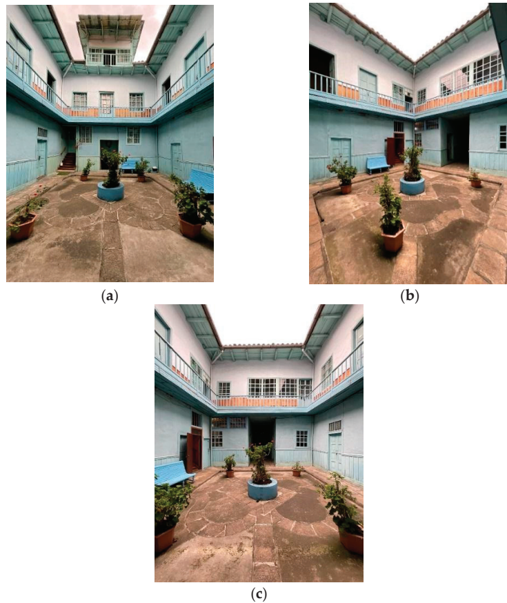
Figure 5. Internal images of the selected building for the study. (a) west facing gallery, (b) galleries facing the main street and north, (c) gallery facing the main street.
