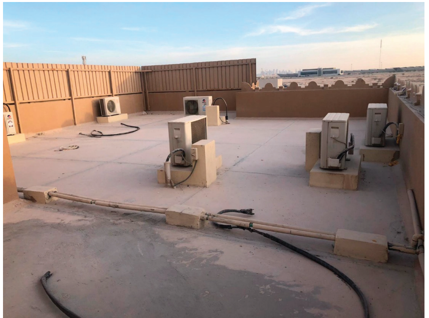
Figure 5. Example of a surveyed home roof.
