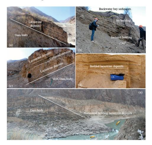
**Figure 13.** Typical geological phenomena. (**a**) Inclined lacustrine sedimentary layer on SDX dam body upstream. (**b**) Horizontal sedimentary layer covers inclined sedimentary layer phenomenon on GD dam body. (**c**) Inclined lacustrine sedimentary layer on SDX dam body downstream. (**d**) Horizontally stratified lacustrine sediments in WDLII-RCR section. (**e**) Horizontally bedding lacustrine deposits layer on RCR dam body upstream.
