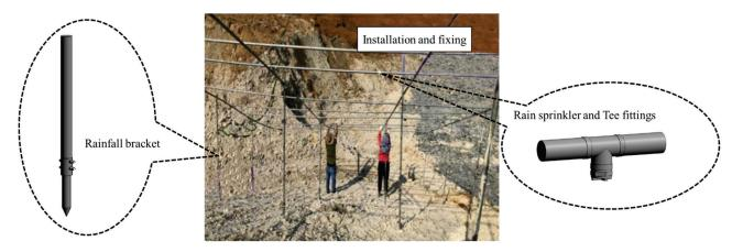
Figure 6. Site installation of the rainfall system.
