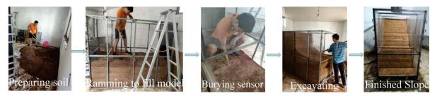
Figure 5. Slope model construction process.
