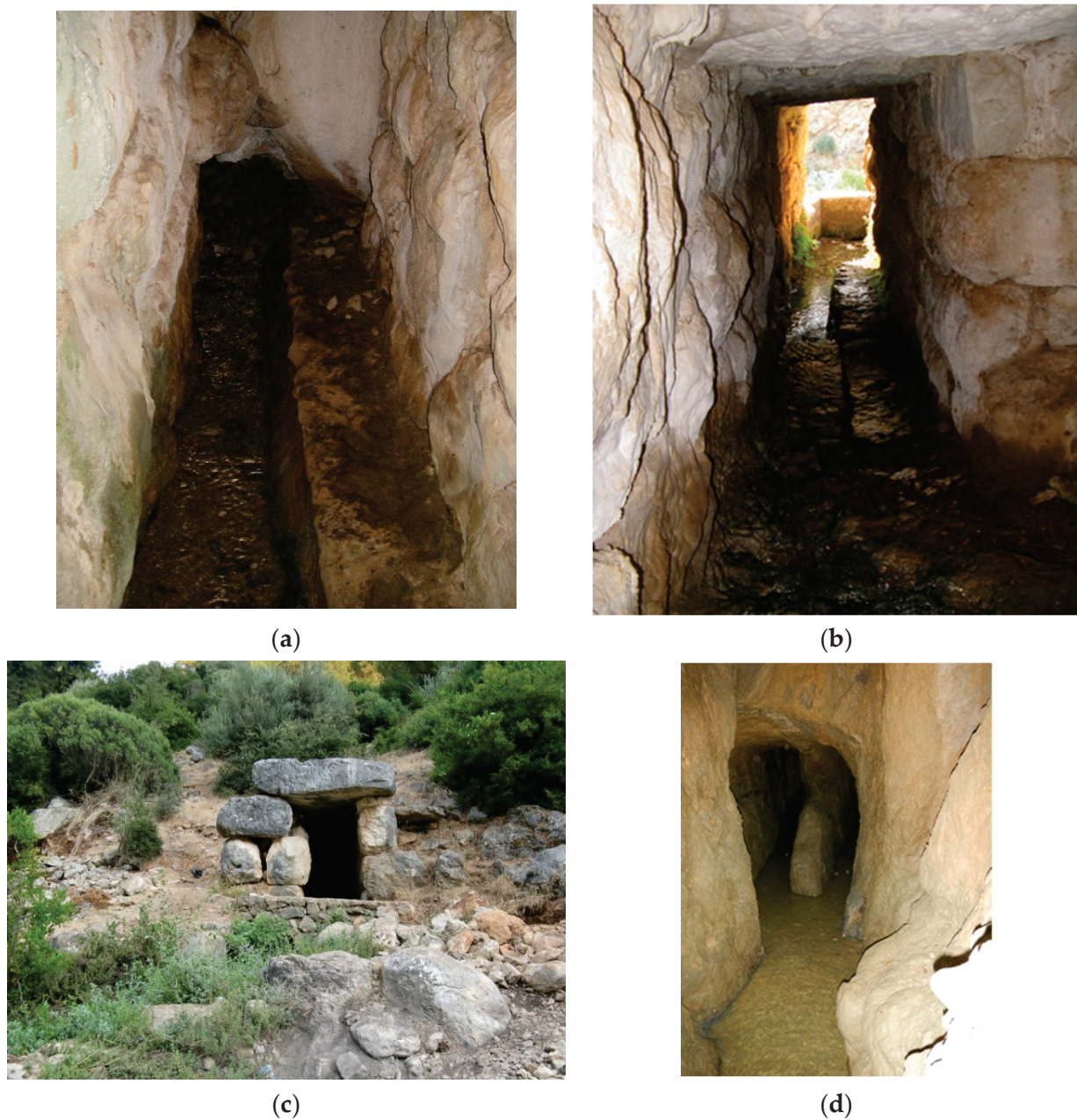
Figure 12. Spring tunnel of the Xanthos aqueduct, Turkey. The tunnel was partially dug into the rock and extended with ashlar and cover stones. The channel is deepened, leaving a footpath along the side for access: (a) inside, looking to the exterior; (b) inside, looking towards the spring; (c) exterior. The structure is still in use to provide water for irrigation. (d) Branching tunnel of Novalja, Croatia. The tunnel was bifurcated to access two springs (Photos Cees Passchier).
