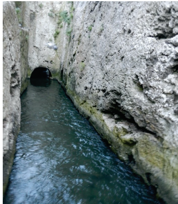
Figure 19. Tagliata Etrusca, Ansedonia. A tunnel and gallery cut into the rock to modify currents in the harbor of Cosa, meant to avoid silting (Photo Cees Passchier).
