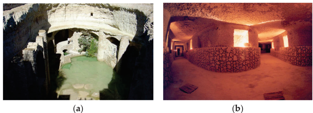
Figure 2. The Kish qanat: (a) the appearance and (b) view of the main tunnel.
