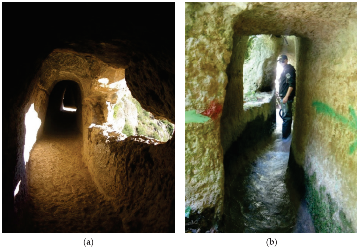
Figure 18. Valley-side tunnels with “windows” from which the tunnel was excavated: (a) Chaves aqueduct, Spain, and (b) Galermi aqueduct, Sicily (Photo Cees Passchier).
