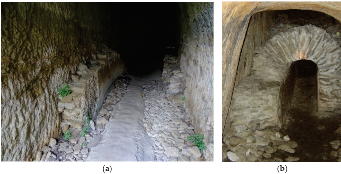
Figure 16. Conduits built into an aqueduct tunnel: (a) Sernhac tunnel, France; a masonry channel was built into the tunnel for passage of the Nîmes aqueduct (Photo (a)—Cees Passchier). (b) Cave de Curée, with a vaulted aqueduct channel in the tunnel, part of the Gier aqueduct of Lyon, France—( http://www.romanaqueducts.info/ , accessed on 15 August 2023).
