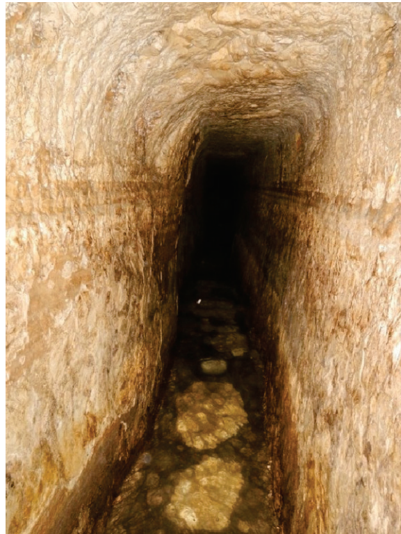
Figure 7. Hezekiah's tunnel. This tunnel still carries water (Photo Cees Passchier).
