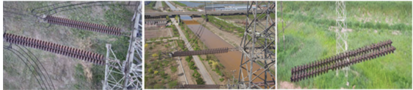
Figure 2. Aerial images of insulators on different backgrounds.
