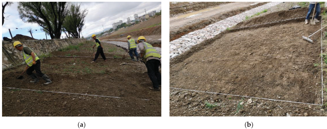
Figure 7. Site preparation: (a) slope preparation; (b) the slope after preparation.
