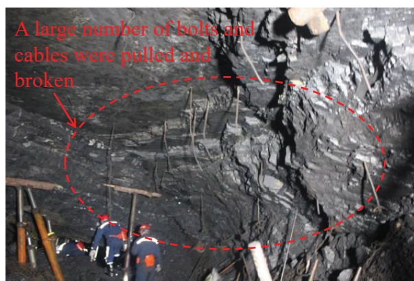
Figure 3. Photo of the anchor bolt (cable) breaking.
