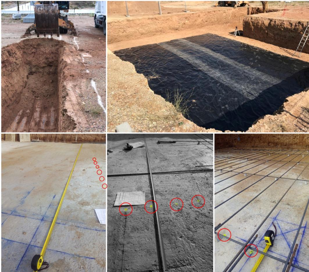
**Figure 15.** Image showing the process of building stakeout before excavation with gypsum, slab perimeter stakeout on polyethylene film with spray coupled to DRON; marking pillars with a traditional shape strip and reinforcement of the foundation slab with dotting of slab rebar by UAV and spray. The different processes show the difficulties in marking the lines executed with a computer in the field.
