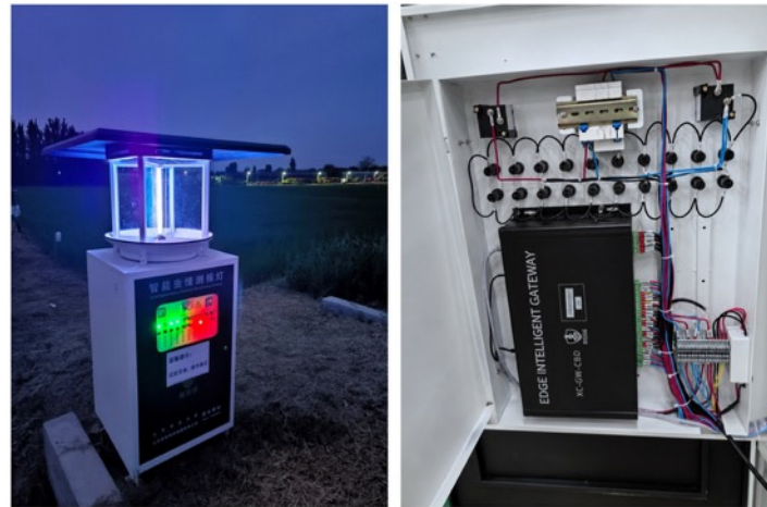
Figure 13. Test site and installed equipment. The Chinese inscription on the front panel identifies the unit as an “Intelligent Insect Monitoring Lamp”. The warning label reads “Notice: Experimental equipment, please keep away.” The device was manufactured by Shandong Xiangchen Technology Group Co., Ltd. (Jinan, China).
