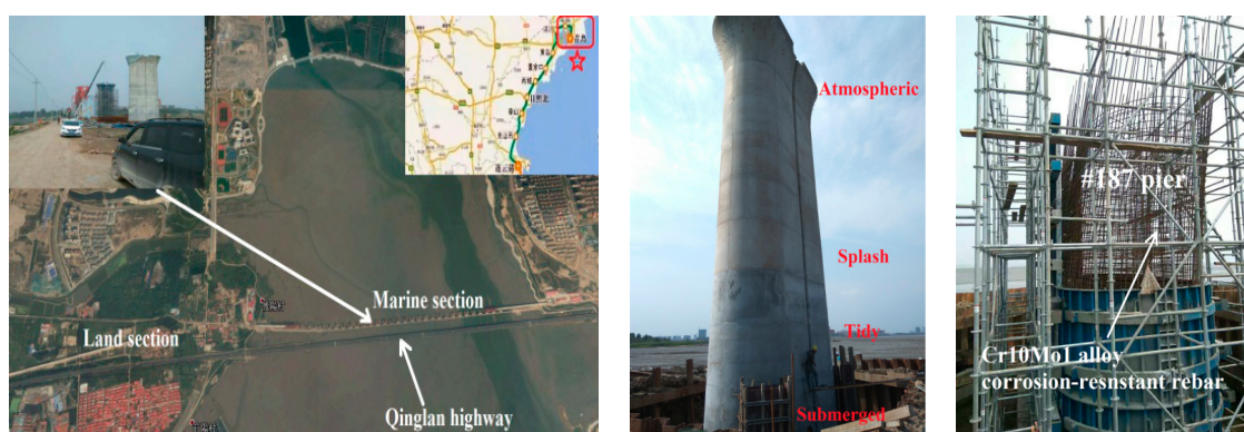
Figure 1. Reinforced concrete pier of the Jiaozhou Bay sea-crossing railway bridge (marine section).
