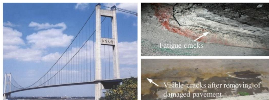
Figure 1. Fatigue cracks in the Jiangyin Yangtze River Bridge.
