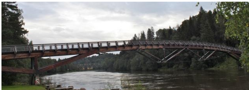
Figure 9. The Lardal footbridge. (Picture after http://broer-vestfold.blogspot.com/2011/08/bro-v-kjrra-fossepark-i-lardal.html ).
