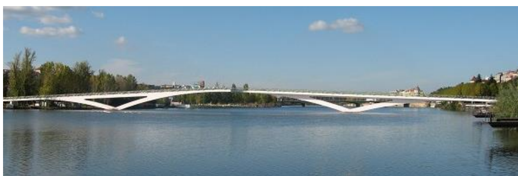
Figure 8. The Pedro e Inês footbridge. (Picture after https://structurae.net/en/structures/pedro-and-ines-bridge ).
