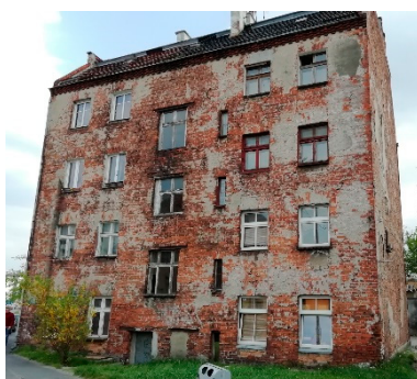
Figure 1. The example of the analyzed tenement house.
