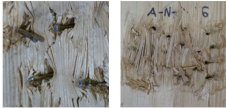
Figure 12. Damage to CLT vertical panels due to embedding.
