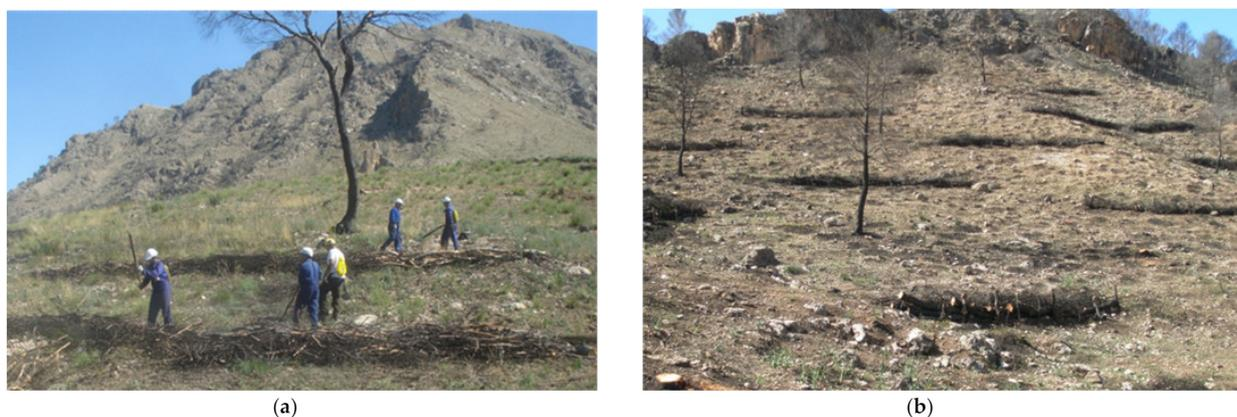
**Figure 3.** Photos of the construction of contour-felled log debris (a) and log erosion barriers (b) in Sierra de los Donceles forest (Castilla La Mancha, Spain).
