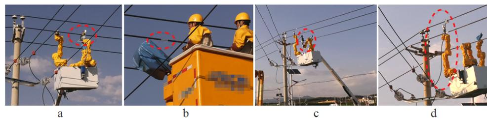
**Figure 24.** Field work: drainage operation on overhead lines. ((a) wire stripping, (b) inspect stripping quality, (c) install the clamp, and (d) single-phase drainage operation is complete).
