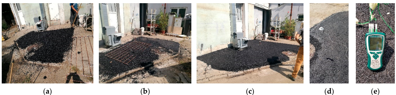
Figure 2. (a) Support layer uniformity; (b) incorporation of copper register and coating with 5 cm of BA8 asphalt; (c) stand after compaction; (d) monitoring of solar radiation level with Ahlborn Star Pyranometer FLA 628 S; (e) monitoring of temperatures with Ahlborn acquisition station and K-type thermocouples.
