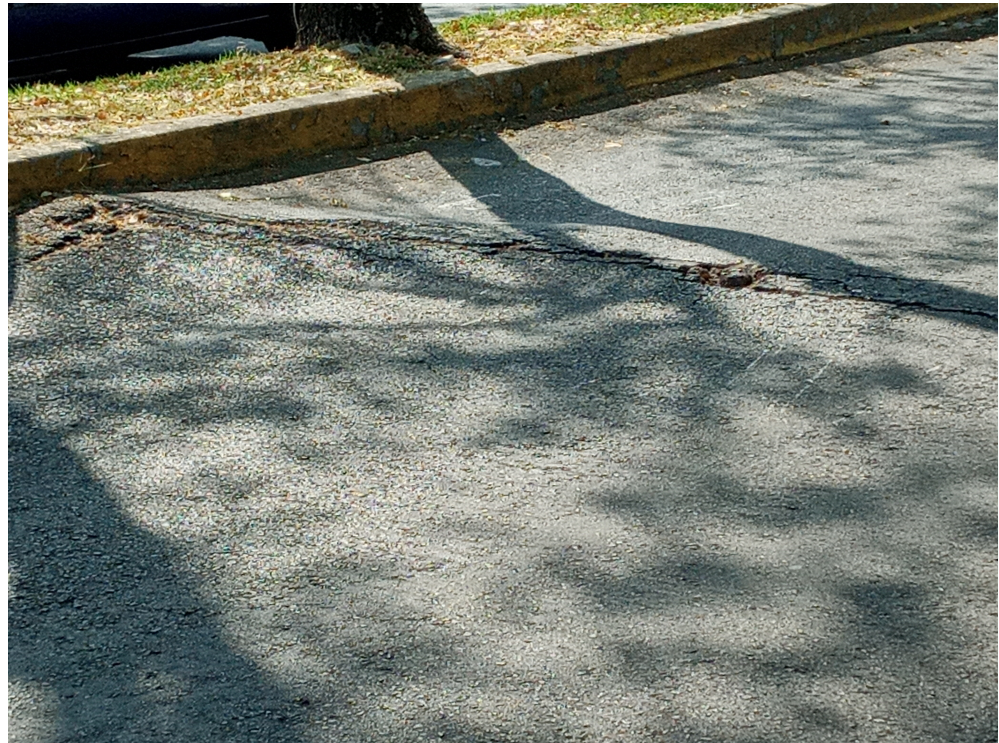
Figure 3. Somewhere in Mexico City. This is an example where a pothole turns into a “speed hump” caused by tree roots. Observe the sinking/uplift region.
