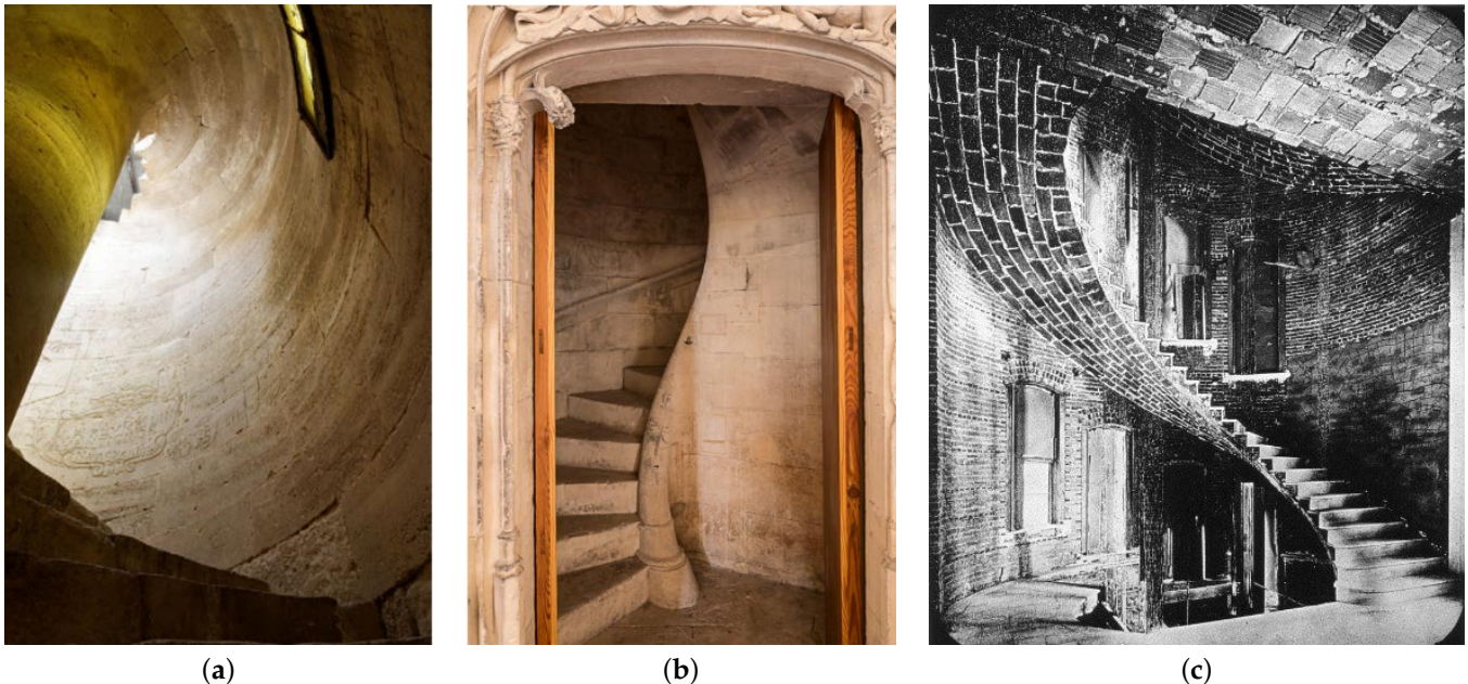
Figure 1. (a) Interior view of the vis de Saint Gilles in Languedoc (France). Notice the inscriptions made by 17th-century stonemasons on the walls of its perimeter box. (b) The spiral staircase of the northwest tower of the Lonja of Palma de Mallorca (Spain). (c) Guastavino helicoidal tile stair in the First National Bank of Peterson, New York City, ca.1890 (Guastavino archive, Columbia University) .
