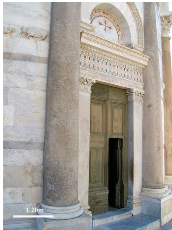
Figure 2. Columns of Giglio granite at the base of the Pisa Bell Tower.
