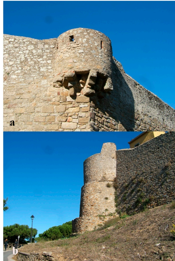
Figure 3. Giglio Castello: walls of the 16th century, built with granite ashlar (a). Giglio Castello: detail of a tower of the city walls resting on a granite outcrop (b).
