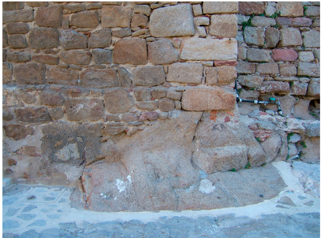
Figure 5. Detail of a granite ashlar masonry in which the intense chromatic alteration is evident (the rock changes from an overall grey colour to a "rust" colour) and the strong intergranular disintegration.
