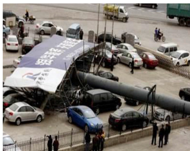
Figure 2. Typical failure in the support of single-post large billboards. Source [4].
