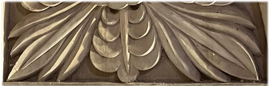
Figure 5. Detailed view of the finishing work on the lime wood implemented by wood-carvers' handiwork.
