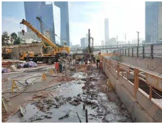
(a) Excavation Initial (26 November 2018)
