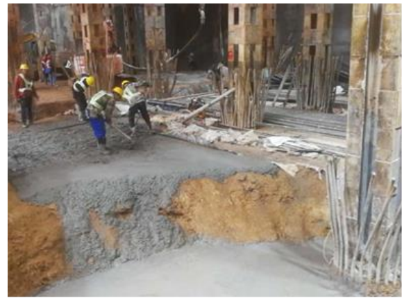
(b) Excavation to bottom of pit (25 February 2019)
