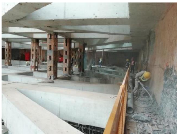
(c) Fifth brace removal (18 March 2019)
