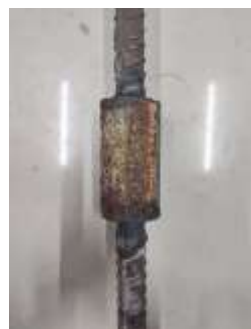
Figure 2. The corroded anchor bolt specimen.
