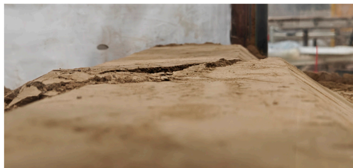
Figure 15. Subgrade settlement.
