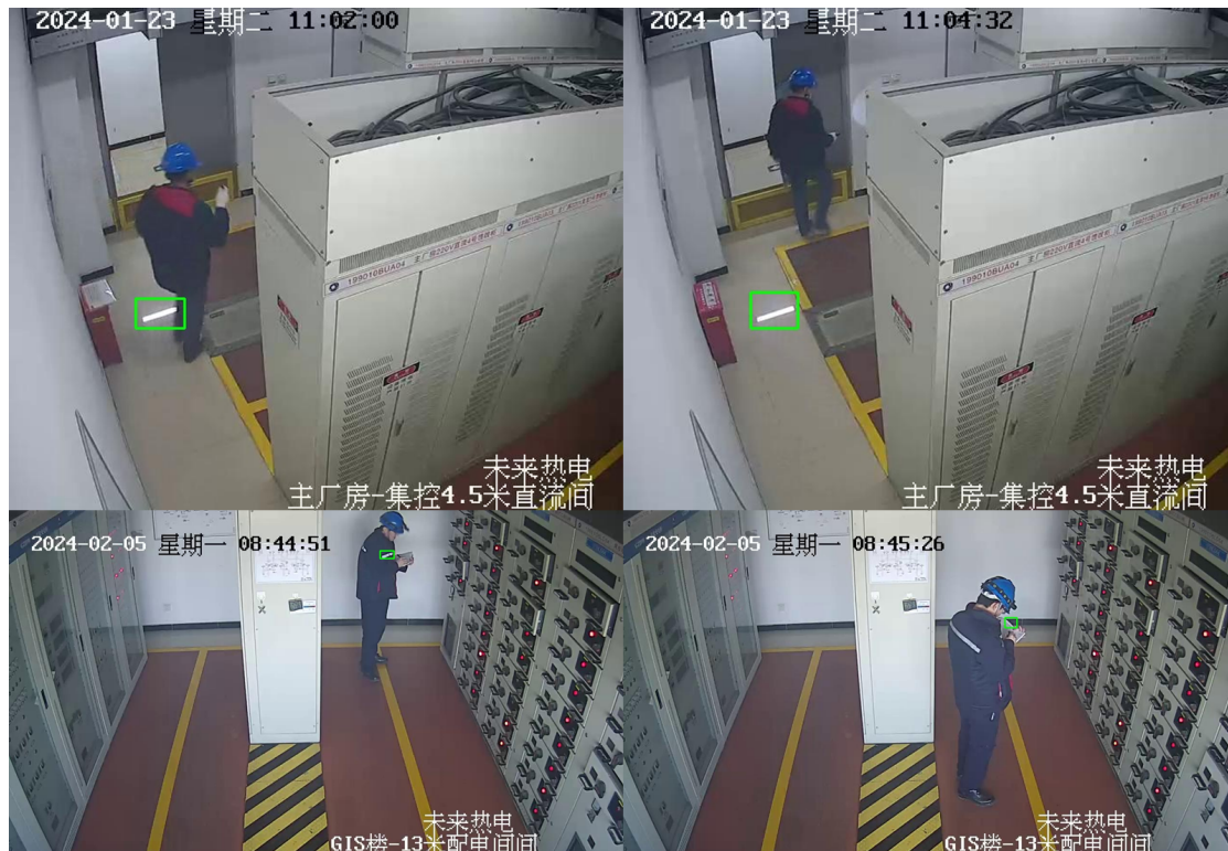
Figure 16. False positive of smoking. These four images are all from the Central Control Room (Upper). Due to various reasons, some types of images may be misidentified. In particular, the image in the bottom right corner could also be mistaken for smoking by human eyes.
