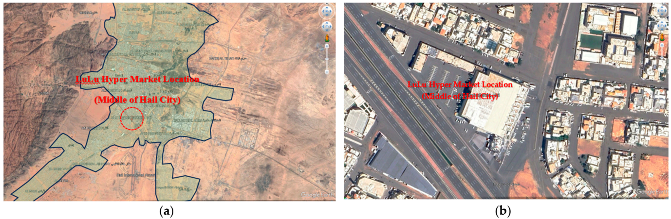
Figure 4. LuLu's Hypermarket location (a), and plan view before the PV unit installation (b).
