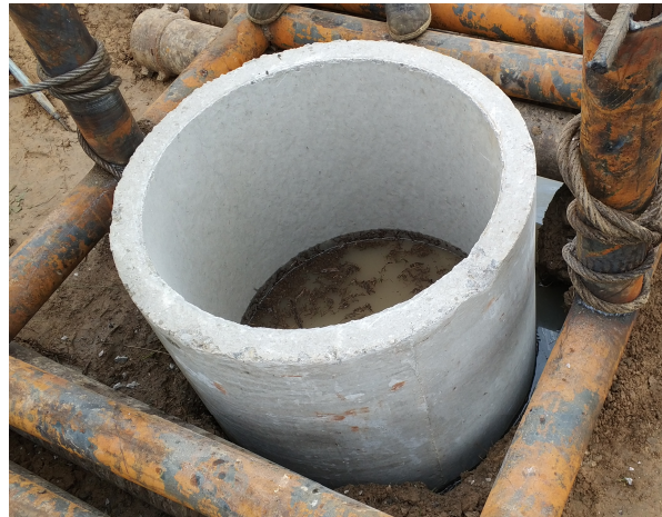
Figure 3. Concrete wall-protective pipe.
