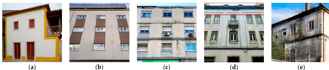
Figure 3. Levels of severity of stains/colour changes in painted façades: (a) Level 0; (b) Level 1; (c) Level 2; (d) Level 3; (e) Level 4.
