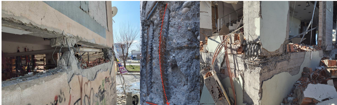
Figure 1. Examples of damage caused by inadequate transverse reinforcement.
