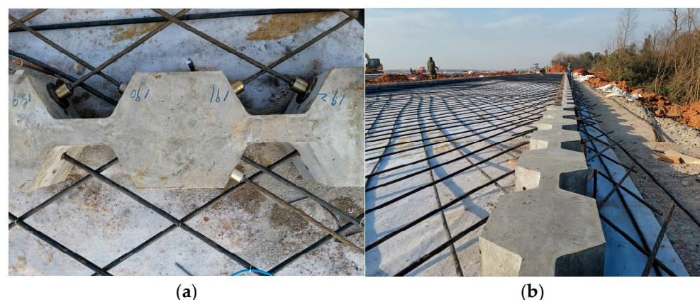
Figure 7. PIA device used in test site: (a) after placing prestressing tendons; (b) after the assembly process.
