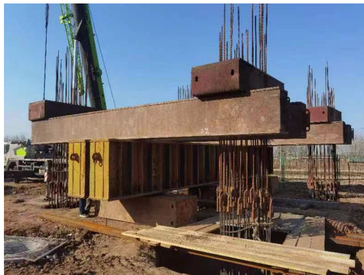
Figure 8. On-site bearing capacity test.
