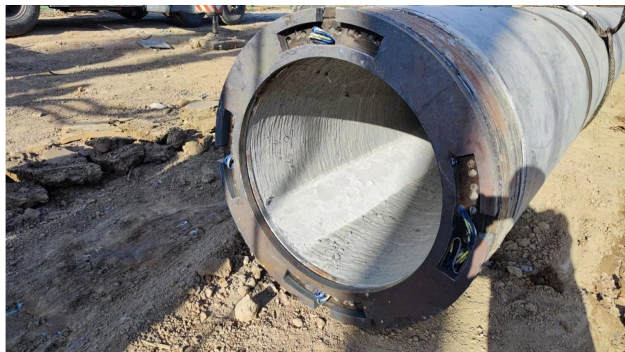
Figure 3. End plates for PHC pile connections.
