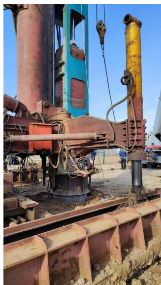
Figure 5. Hydraulic-hammer pile-driving site.
