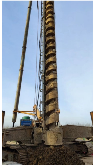
Figure 2. Pre-drilled holes in the test area.
