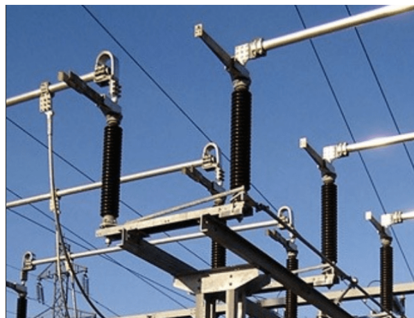
Figure 7. An open disconnector showing the visible isolation gap. Adapted from [25].
