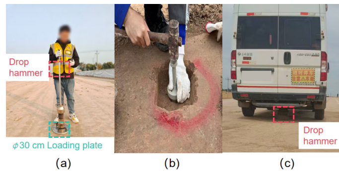
Figure 6. Testing equipment: (a) PFWD; (b) CRM; (c) FWD.
