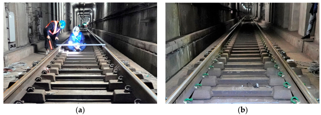
Figure 2. Field survey and overview of the tested tracks for field measurement: (a) field investigation; (b) view of the field measurement section.
