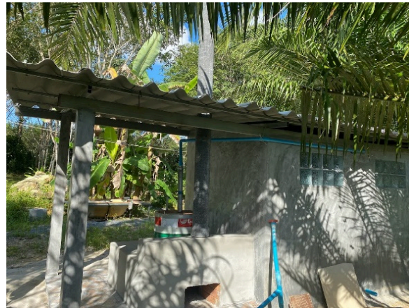
Figure 3. Local stream boiler (control).
